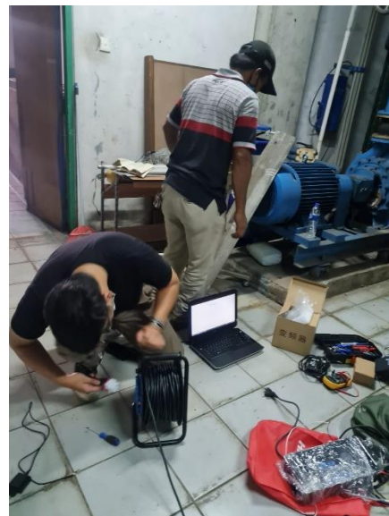
Gambar 4. Instalasi Kabel RS485
